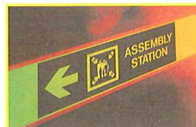
At frequent intervals the low level escape route lighting incorporates an indication of the direction of escape.
